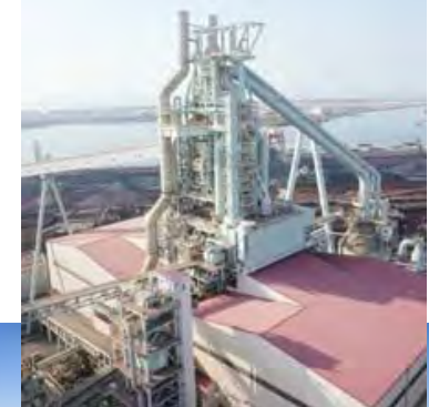
High-rise structure (#2 BF in Wakayama Area)
